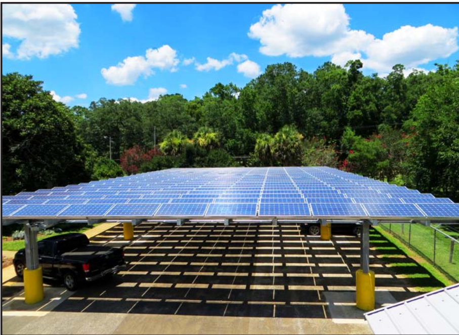
Leon County Net-Zero Facility
